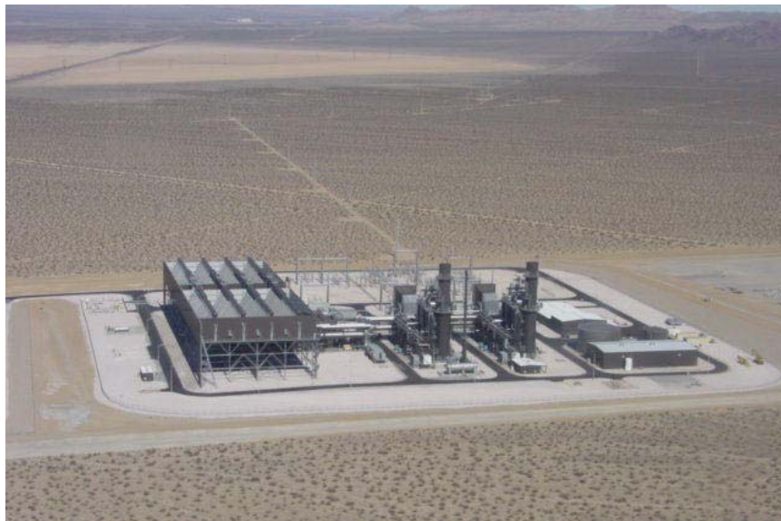
Figure 13 – NGCC Plant with Air Cooled Condenser (Structure to Left)
