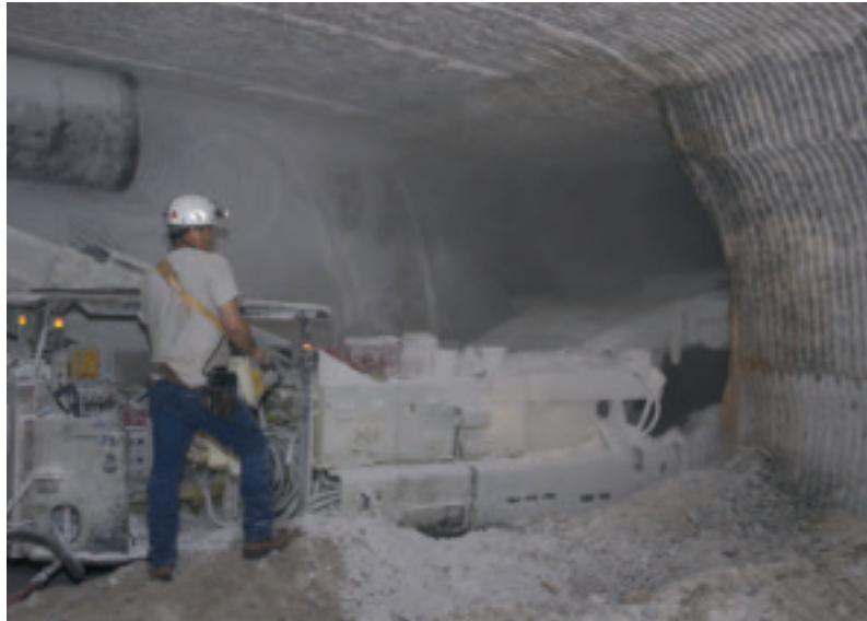
An underground chamber at the WIPP facility.
