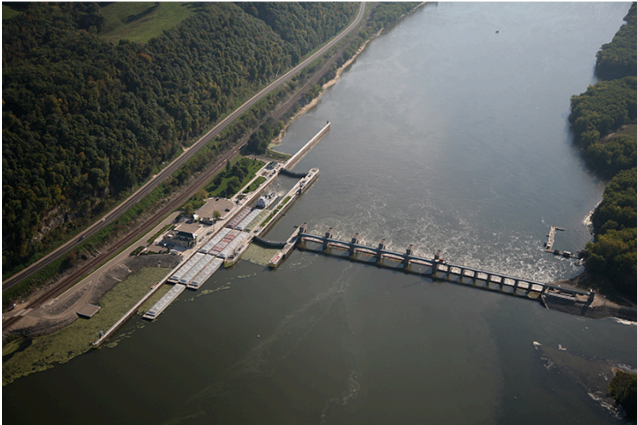
Figure 3.2 (b). Lock and Dam 9 on the Mississippi River near Lynxville, Wisconsin. A similar structure would likely be required on the Missouri River for diversion rates in excess of 6,000 cfs.
