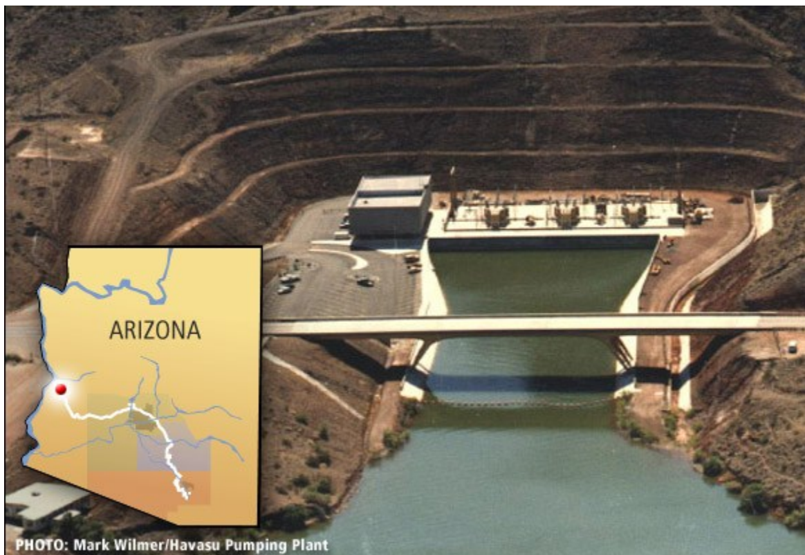
Figure 3.2 (f). Example of a canal pump station from the Central Arizona Project, source www.cap_az.com .
