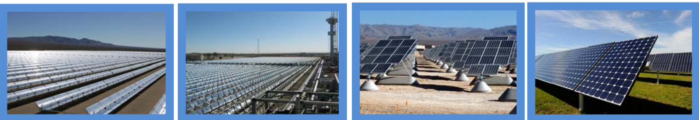
Nevada Solar One
