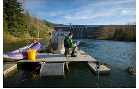
A USACE biologist inspects a fish trap used to help count juvenile salmon migrating below Lookout Point Dam in the Willamette Valley. Adjusting the operations of dams can improve water quality and habitat for fish and wildlife and meet ongoing human needs. Credit: ©Bridget Besaw 2008
