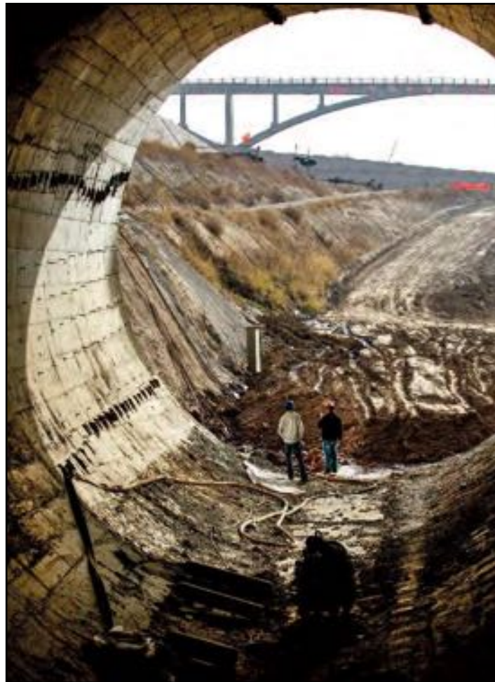
Circle of Blue, as part of an investigation of the extensive manmade river that will move water from central China to Beijing, captured views of the massive infrastructure of the South North Water Transfer Project, like this aqueduct under the Yellow River.
